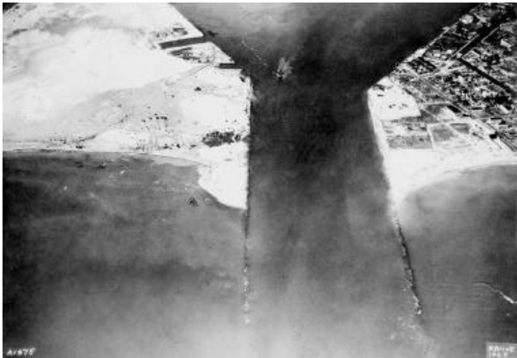
Figure 21. Aerial view Bakers Haulover Cut after the Hurricane of 1926 (December 1, 1927). (See Figure 12 for aerial photograph of bridge before the hurricane. Biscayne Bay is at the top of the image and Miami Beach is at the bottom. Note erosion of the sides of the Cut. Bridge destroyed during the hurricane has been removed.) [R. B. Hoit, photographer. Photo negative, black and white, 4 x 5 in. N035203 . General Collection, Florida State Photo Archive. < http://fpc.dos.state.fl.us/ >]
