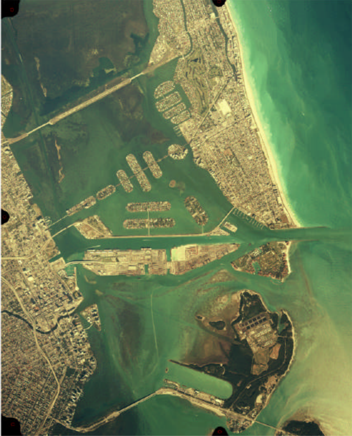
Figure 36. Central Biscayne Bay. [Some of the channels, such as the one between the Miami River and the Virginia Key Sewage Treatment Plant can be observed. The left-most rectangular indentation in the Port of Miami was home base to NOAA and University of Miami research vessels. The deep area north of the 36th Street Causeway is the dark colored area. Note seagrass bed at the top left of the image.] [Aerial photograph 5WGQ2987, 1992. Scale 1:48000, azimuth 191.1, 25.76833° N, 80.14556° W. (Coastal Aerial Photography, NOAA/National Ocean Service, < http://mapfinder.nos.noaa.gov:80/mapfinderhtml3/surround/photos/photos.html >, < http://mfproducts.nos.noaa.gov/images/Photos/5WGQ2987.gif >. Black areas are artifacts in original photograph. See Figure 2 for identification details.] See color version on p. 119.
