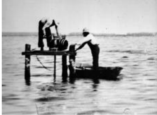
Figure 8. Mariners installed a pipe and built a platform to make water from a fresh spring in Biscayne Bay. [Photograph 117D. Munroe Collection, Historical Association of Southern Florida.]
