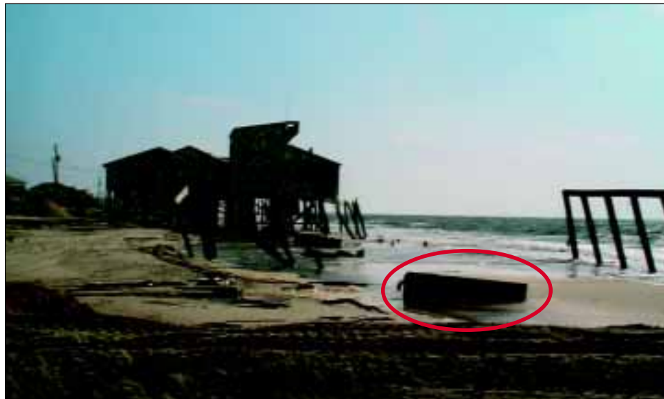
FIGURE 4-19 Old concrete septic tanks (circled) and drain fields have been superseded by the new municipal sanitary sewer system. The old systems still create a hazard as waterborne debris.
