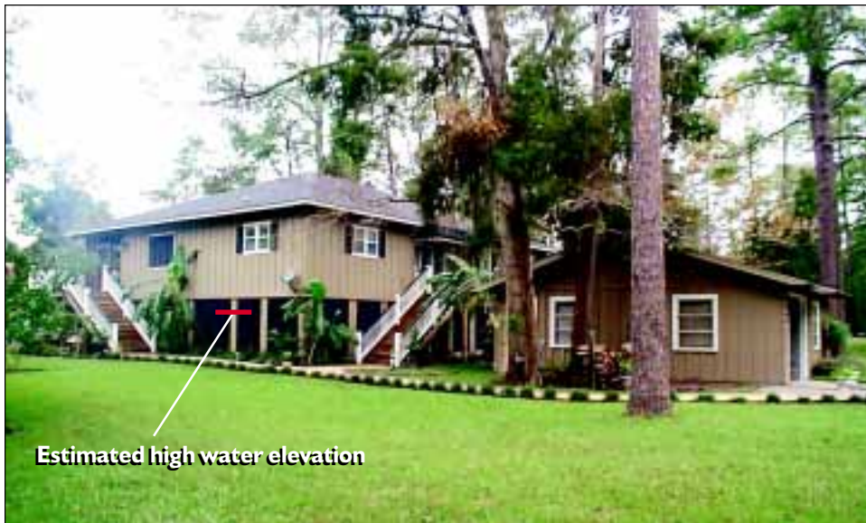
FIGURE 4-5 House along the Fish River, elevated through FEMA's HMGP that suffered minimal flood damage.
