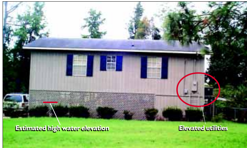
FIGURE 4-6 Previously elevated house along the Fish River suffered damage to contents below the first floor. Note that the homeowner also elevated utilities on the right side of house, preventing loss or damage.
