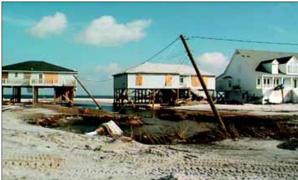
FIGURE 4-35 Utility poles damaged by wind, coastal surge, and erosion.
