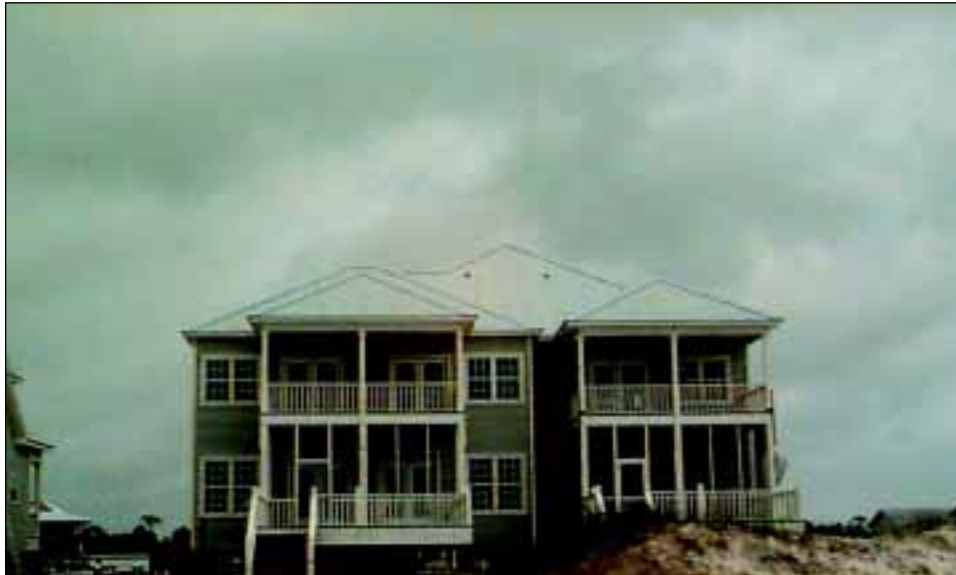
FIGURE 4-38 Metal roofing system on multi-family building in Fort Morgan performed well.
