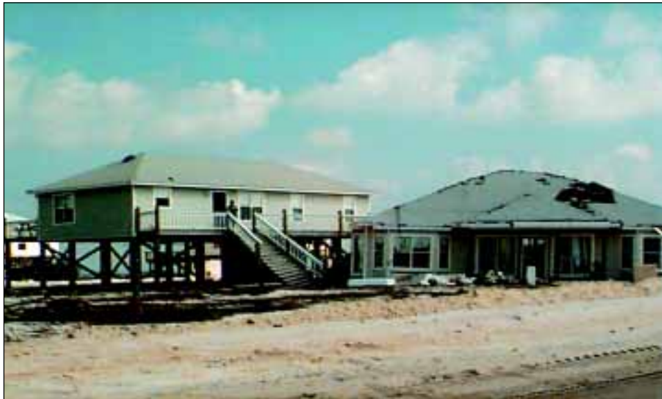
FIGURE 4-10 The structure on the right lost its pile foundation system and was washed into the structure on the left.
