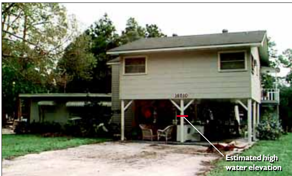
FIGURE 4-2 Approximately 5 feet of flooding at this house along the Fish River caused no damage to the elevated addition.
