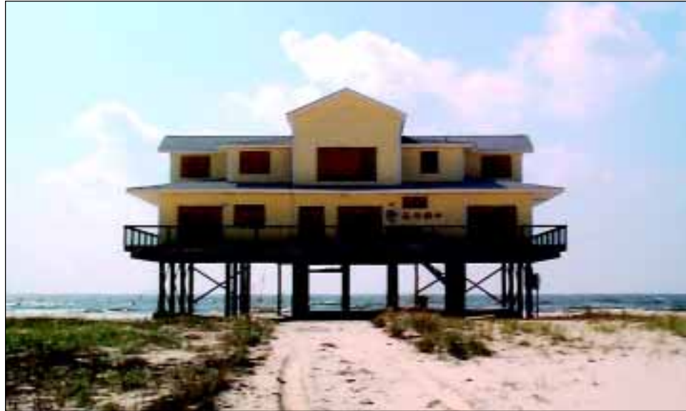
FIGURE 4-18 This house sustained no damage with the exception of loss of stairs and items stored below the first-floor elevation.
