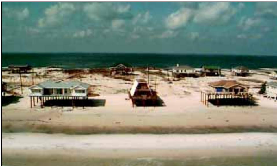
FIGURE 4-37 Fully exposed front-row houses that exhibited minimal wind damage.
