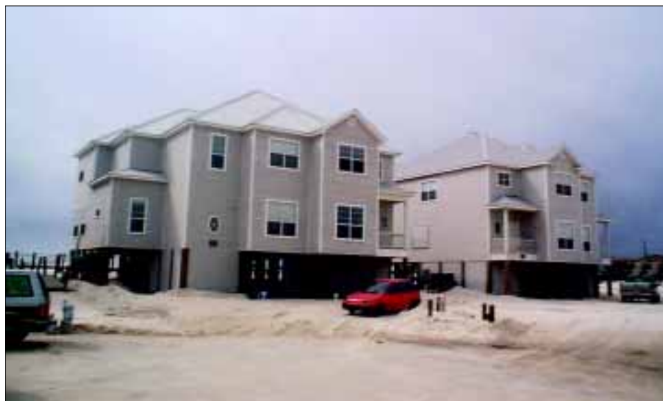
FIGURE 4-26 These multi-family buildings in Fort Morgan suffered no damage from coastal storm surge. Proper elevation, siting, and building materials contributed to their success. Note roof design that minimizes the use of gable ends.
