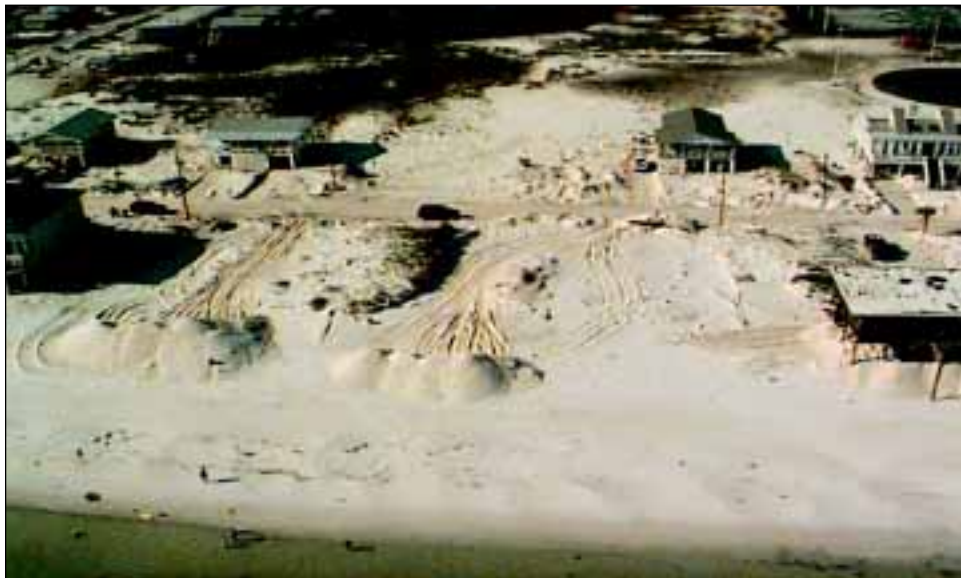
FIGURE 3-9 Sand accumulation from overwash in Pensacola Beach, Florida.
