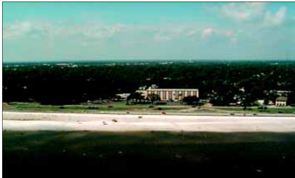
FIGURE 3-5 Mississippi Gulf Coast near Biloxi. Minimal coastal surge damage or overwash was observed.
