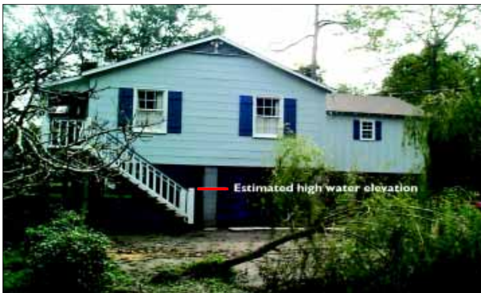
FIGURE 3-3 Elevated home along the Fish River in Baldwin County, Alabama, that received minimal damage.
