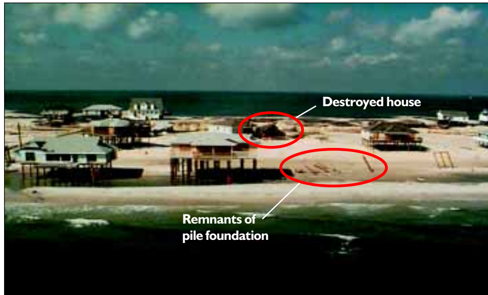
FIGURE 3-4 Front-row house separated from its foundation and destroyed by the storm on Dauphin Island, Alabama. Note the properly elevated and set back house on the right fared very well.
