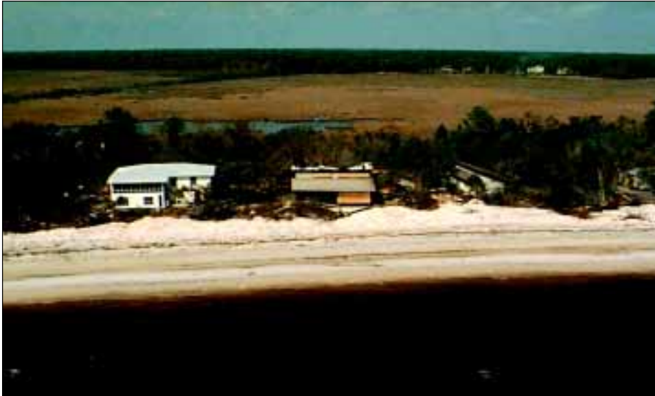
FIGURE 3-6 Overwashed sand accumulation and minor structural damage near Gautier, Mississippi.
