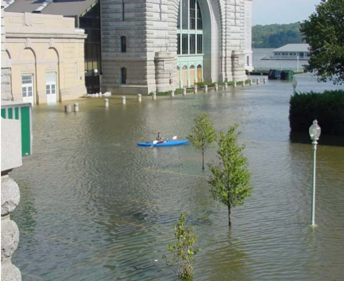
Picture 4. Storm surge flooding from Isabel at the U.S. Naval Academy in Annapolis, MD. Courtesy of U.S. Naval Academy Public Affairs.
