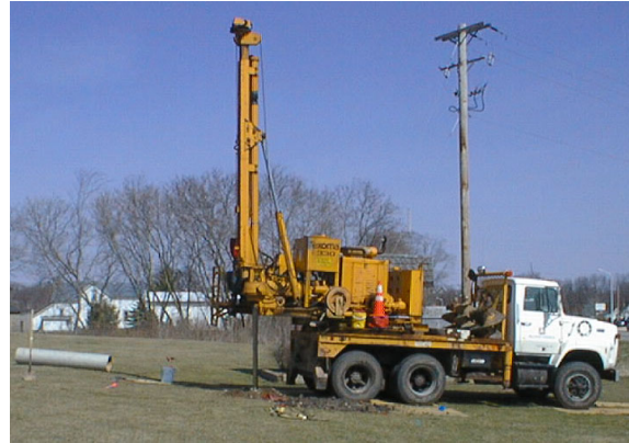
Drilling Hole for a Concrete Post
