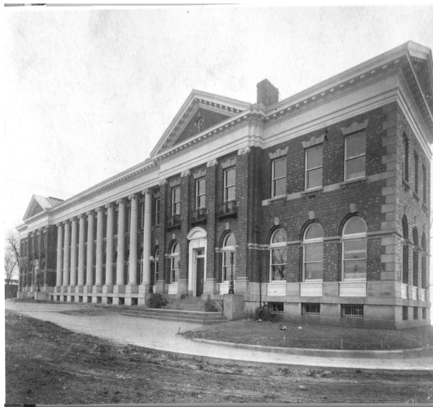
Building at 25 th and E Streets, NW Office of NIH History
