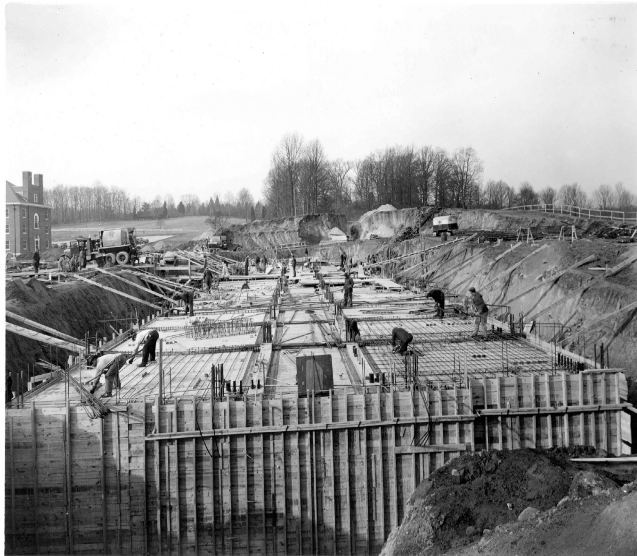
January 1939: Building 6's foundation.
