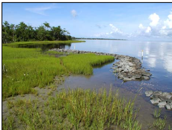
Living shorelines, such as the restored marsh and low rock sill in North Carolina, can be used to address shoreline erosion.
