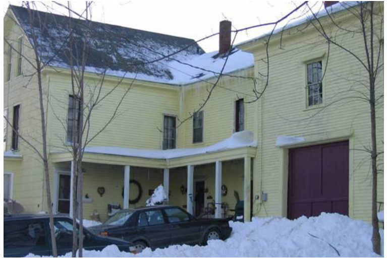
56 School Street, Canton prior to demolition
