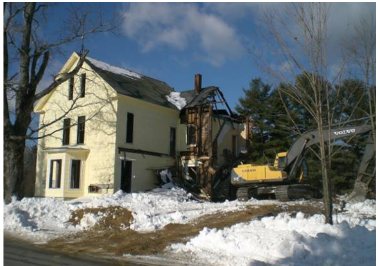
56 School Street during demolition
