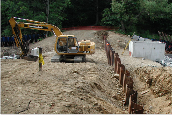
Reconstruction of the dam and outlet control structure, July 2004.
