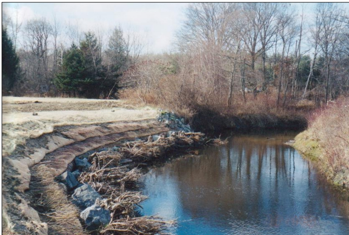
The bioengineered slope along the Mill River after placement in the fall of 2000.
