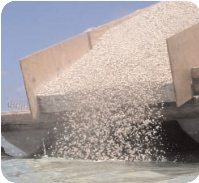
Pearock is poured from a barge to fill a blowhole. Deeper scars and blowholes must be filled because seagrass plants will not grow downward, away from the sun. (Photo: Alicia Farrer)
