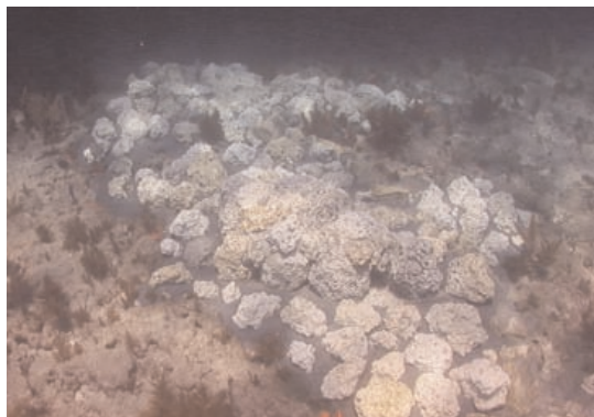
Limestone rocks and concrete were used to build reef modules to fill in large excavations left behind at the site.
