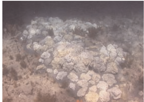
Limestone rocks and concrete were used to build reef modules to fill in large excavations left behind at the site.
