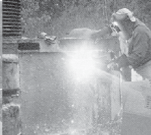
A welder used a high-tech torch to cut through the bottom plate of the pump to remove cocaine packages.
