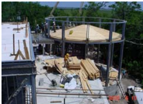
The Magnetic Nuclear Resonance facility was constructed to the specifications of the instruments, ensuring accurate work and less maintenance.
