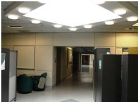
Skylights flood interior hallways, saving electricity. Researchers and other employees prefer the natural light to bulbs.
