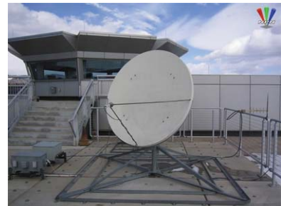
Figure 62. DOMSAT disk connected to the LRGS located on the roof of the David Skaggs Research Center in Boulder.
