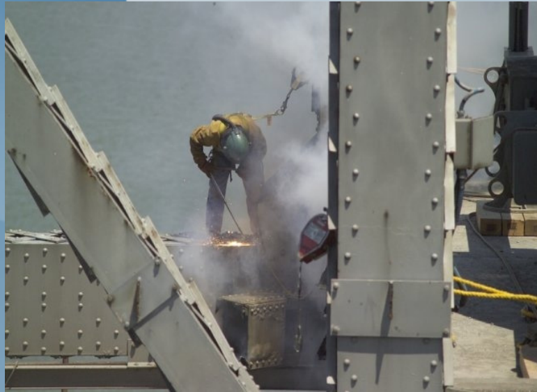
Torch cutting during bridge dismantling
