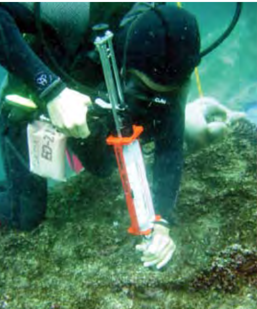
Diver installs mooring buoy in Galapagos. Photo: Amy Massey
