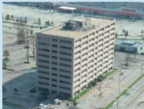
Main office building for the Minerals Management Service, Gulf of Mexico OCS Region. Photo taken September 2005 after Hurricane Katrina.
