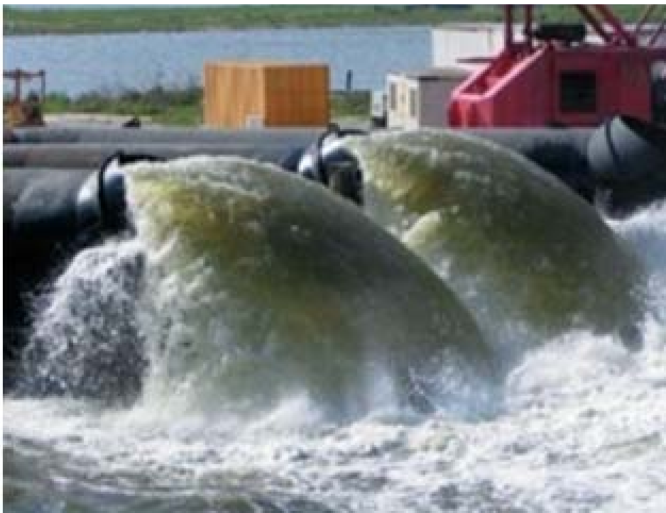
Figure 3-DOD-24. Army Corps of Engineers Working to Protect New Orleans from the Next Hurricane. Pumps at the 17th Street Outfall Canal operate at full capacity during a test on 24 March 2007. Photo by Task Force Hope. (US Army Released)
