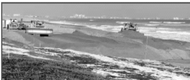
Figure 13: Restoration efforts using OCS sand resources on Patrick Air Force Base near Coca Beach, Florida.
