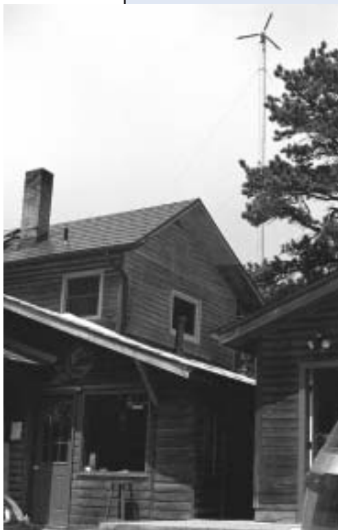
Jim Green, NREL / P1A12796
