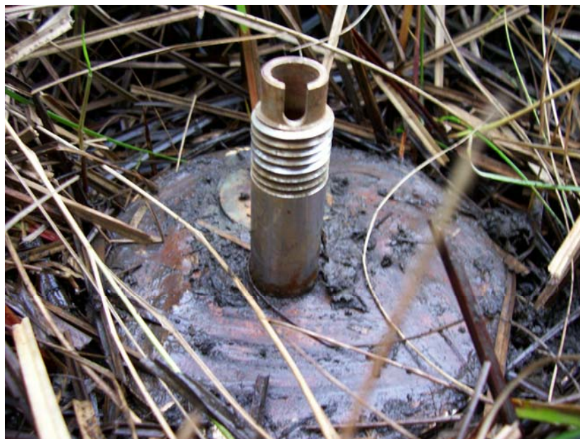
Figure 2.3. BM top type #3 (of 3): Stainless steel receiver with 1"-8 thread stainless steel pipe coupled to a deep-driven, 9/16-inch diameter, stainless steel rod with concrete protecting the coupling from tampering.
