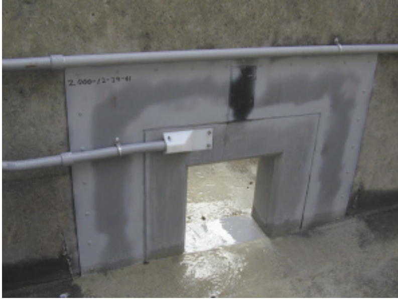
A fish ladder opening with PIT-tag antennas, part of a new detection system for adult salmon. Photo: NWFS.
