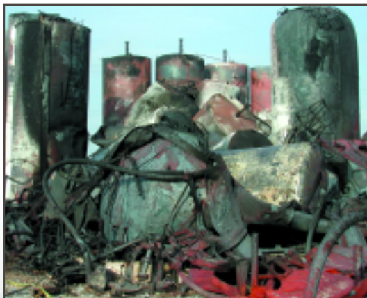
Storage tanks at Third Coast collapsed from the intense fire which burned for over 24 hours.
