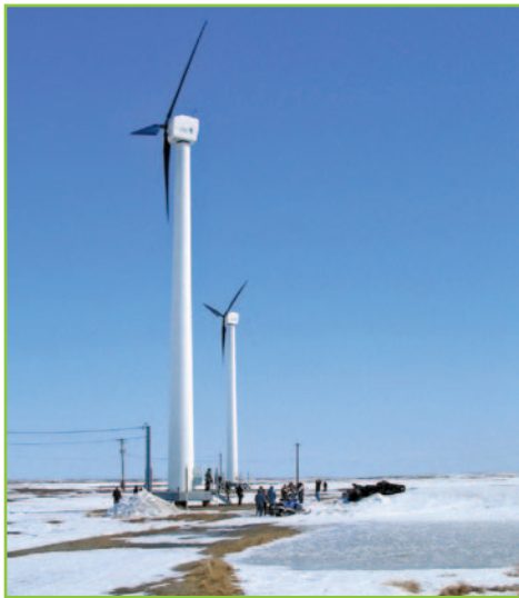
Kasigluk turbines. Ian Baring-Gould/PIX16096.
