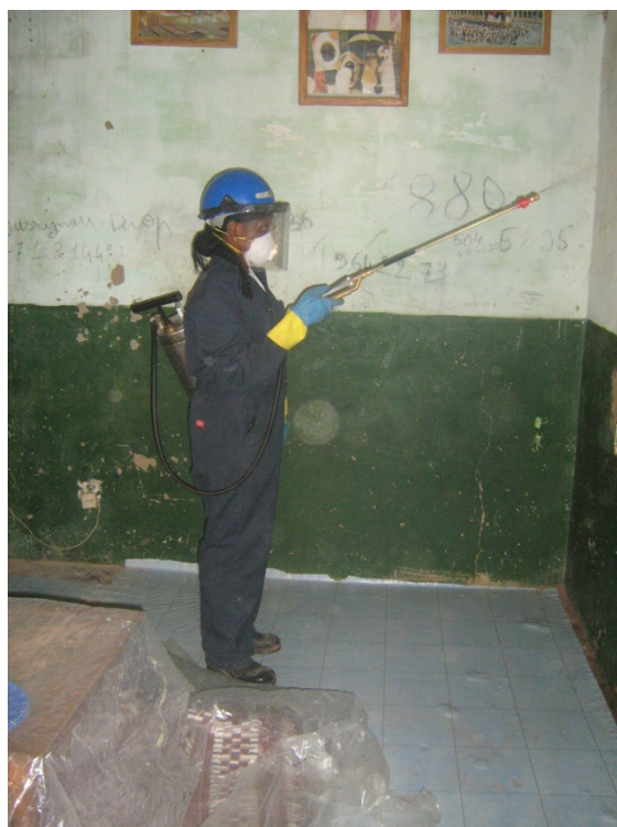
Figure 3. A spray operator at work.
