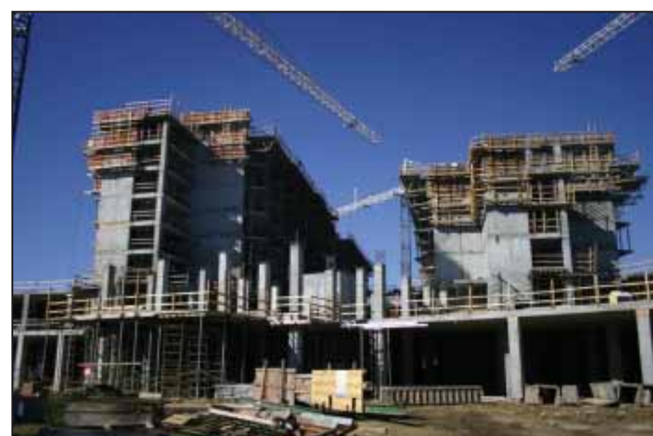
Front of Pavilions A and B.
