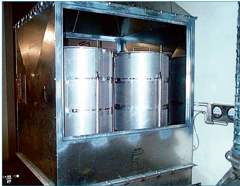
Figure 3-8 A 4,000-cfm filter unit using radial flow filters was selected for the stairwell safe room.
