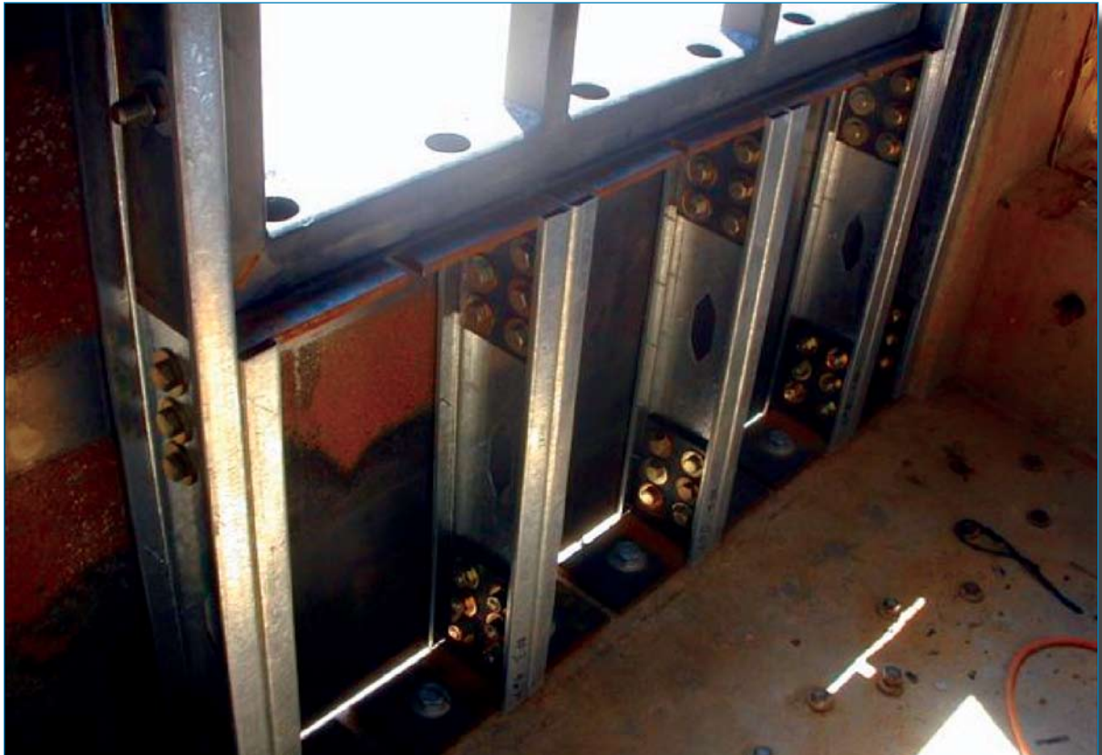
Figure 2-19 Metal stud blast wall
