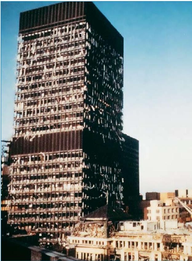
Figure 2-9 Blast damaged façade
