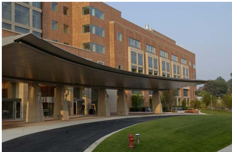
The front entrance to the Mark O. Hatfield Clinical Research Center shortly before its opening in 2005, as evidenced by the presence of a construction worker and lack of the ever present patients, buses and taxis seen today. Since the Clinical Center opened in 1953, clinical research has been a key feature of the NIH intramural research program. Photo courtesy of the Clinical Center.
