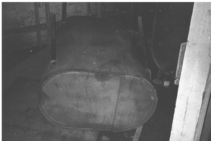
Figure 1.2.1B: Interior fuel oil tank dislocated by buoyancy forces
