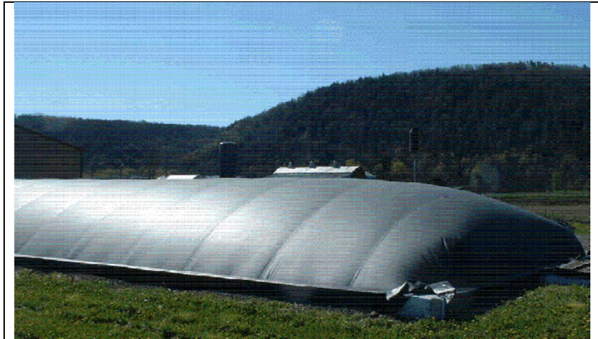
Figure 29 Plug-flow digester. Image courtesy Penn State University 148
