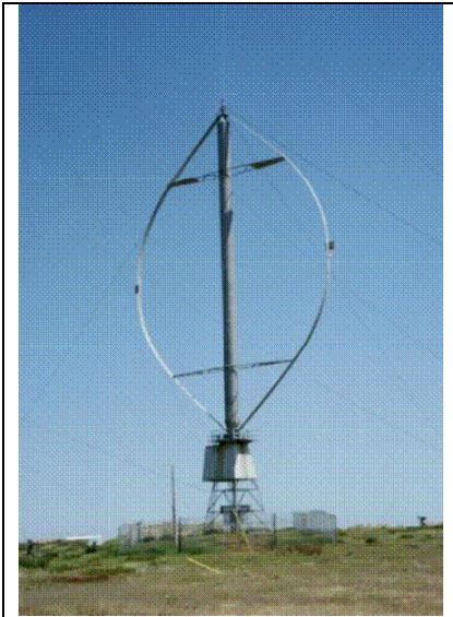
Figure 18 Darrieus style wind turbine. Image courtesy Solcomhouse 80
