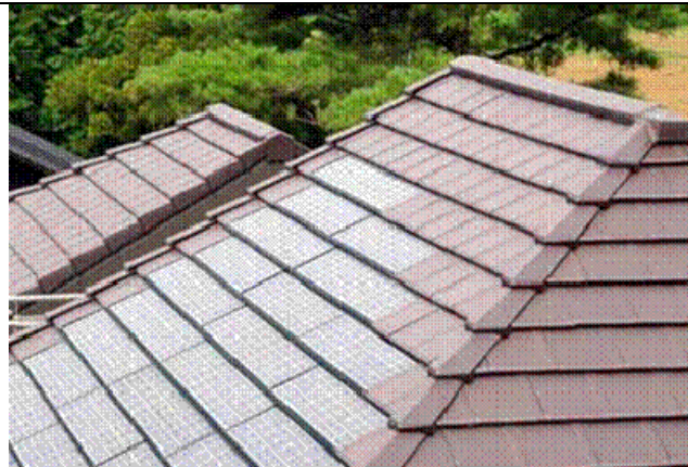
Figure 6 Building integrated PV (BIPV) shingles. Image courtesy Kyocera 38
