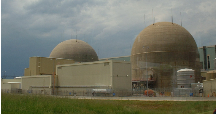
Dominion's North Anna Power Station, in Mineral, VA, offers many career opportunities in nuclear science and technology.
