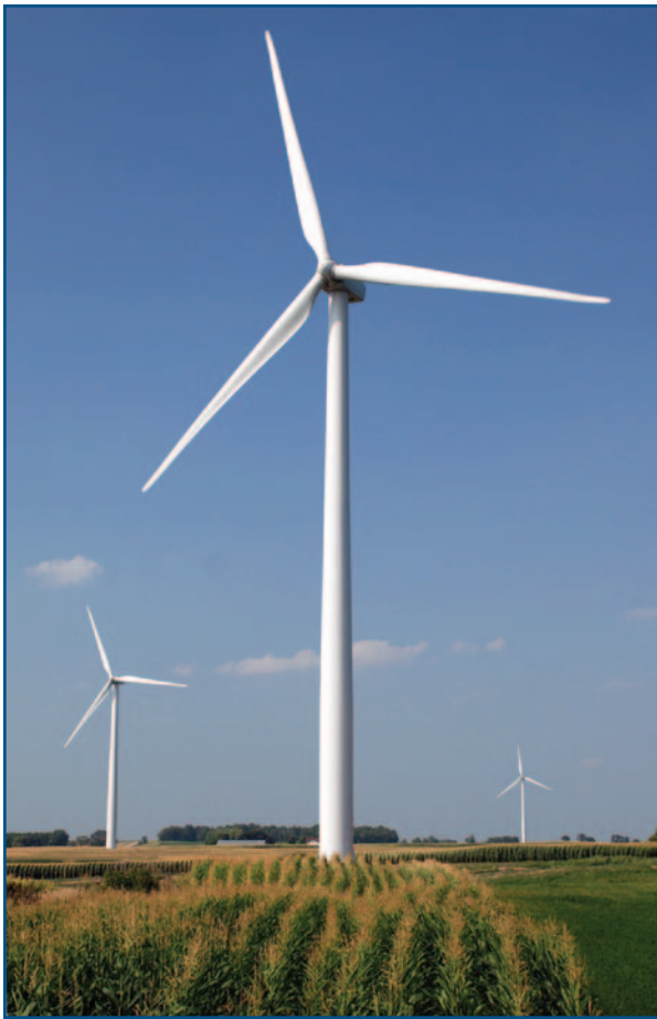
The 129-MW Forward Wind Energy Center in Dodge and Fond du Lac Counties came online in 2008. Invenergy LLC/PIX16037.
