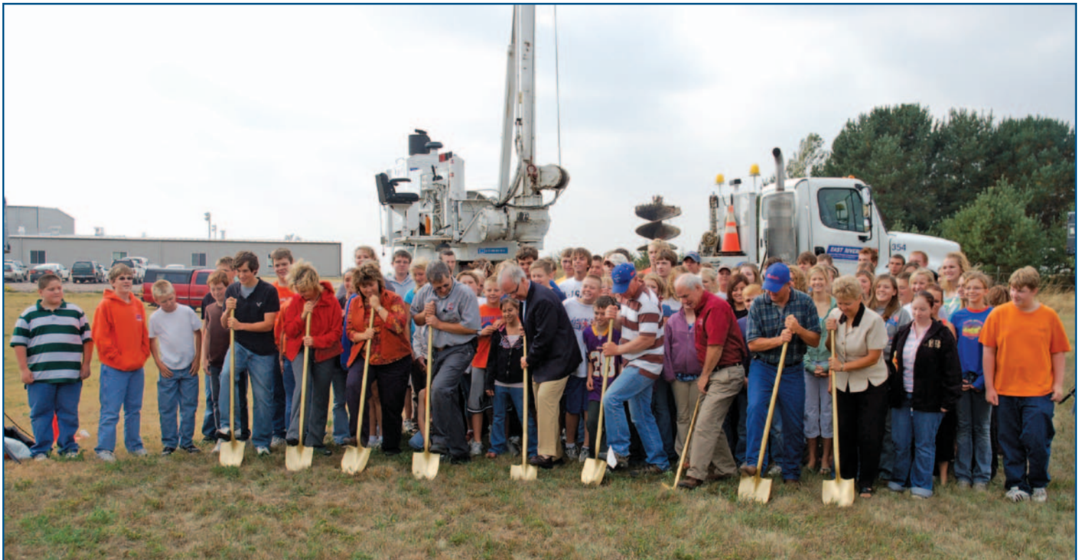
Groundbreaking begins at the Sanborn Central School Wind for Schools Project in Forestburg, South Dakota. Photo credit: East River Electric Power Cooperative.
