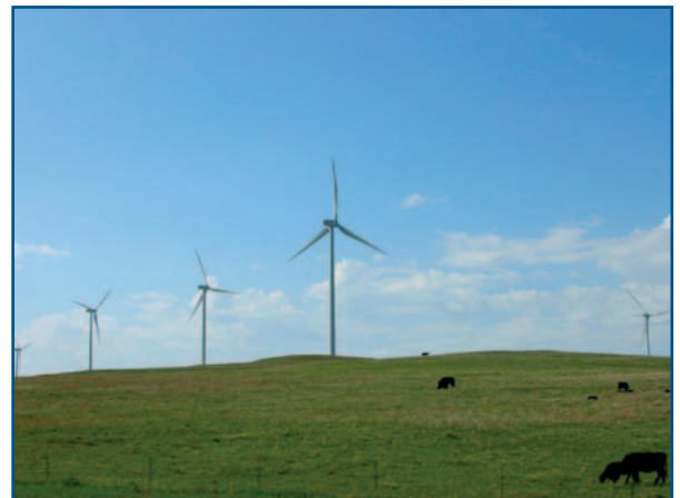
Phase I of the Smoky Hills Wind Farm west of Salina brought 100.8 MW online in Kansas. The completed project will have a 250-MW capacity. Amanda Brown/PIX16023.
