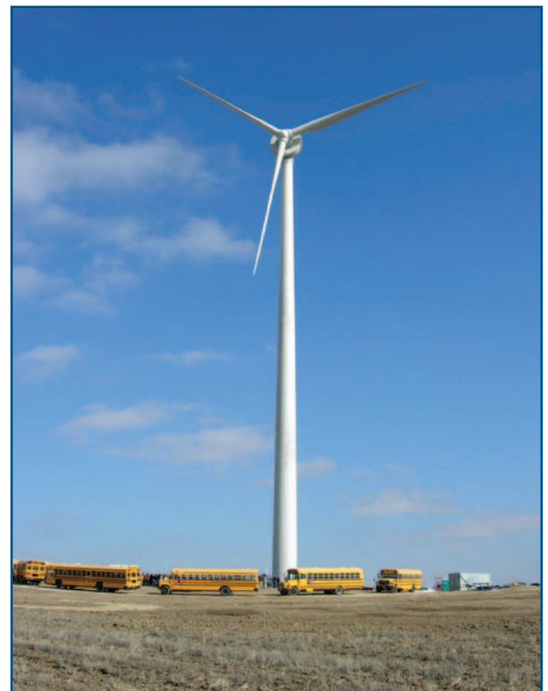
In February 2008, the Wray School District RD-2 dedicated its 900-kW Americas Wind Energy wind turbine. Ian Baring-Gould/PIX15457.
