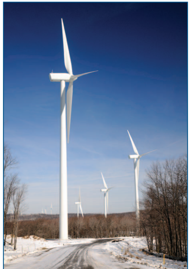
The 164-MW Mt. Storm Phase 1 project came online in West Virginia in 2008. Moe Vetter/PIX16205.
