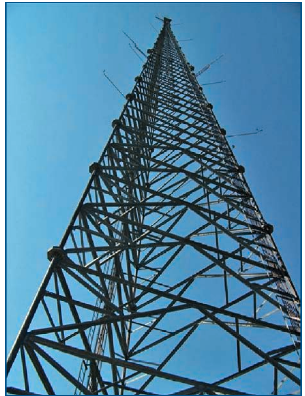
The U.S. Coast Guard (USCG), with assistance from NREL, has been monitoring the wind resource with instrumentation mounted on a 108-m communications tower in Cape May, New Jersey.
