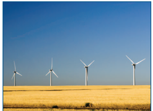
Oregon added to its installed capacity in 2008 with the Klondike III project. Iberdrola Renewables/PIX16112.
