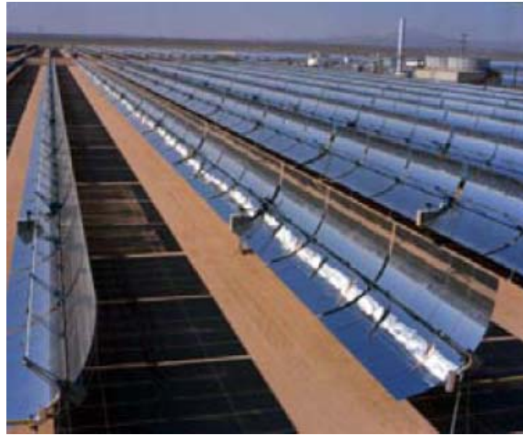
Figure 1.8. Parabolic Trough System
