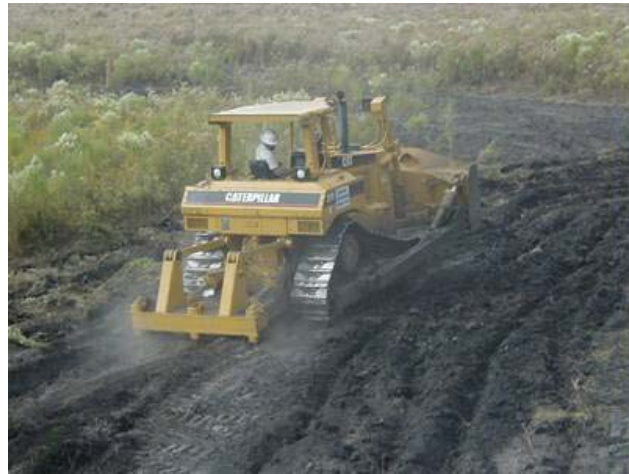
Photo courtesy of Backwater Environmental, Pittsboro, NC.
