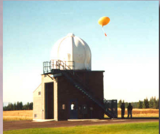
Above: Typical NWS upper air shelter and balloon launch. NWS photo.
