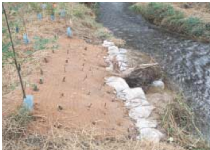
Streambank stabilization projects restore vegetation to stream corridors, reducing stream temperatures and erosion and benefiting aquatic and terrestrial species in the watershed.
