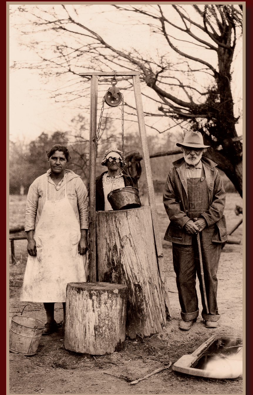
Dug Well with Cypress log as curbing. John D. Locklear and family. Coratan Indians. Robeson County, North Carolina, 1936.
