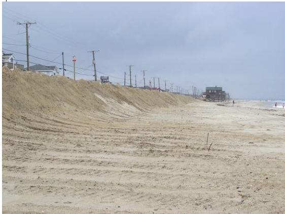
10990 Figure 11.6 Retreat. (a) Houses along the shore in Kitty Hawk, North Carolina June 2002. Geotextile sand 10991 bags protect the septic tank buried in the dunes. (b) October 2002. (c) June 2003 10992 10993
