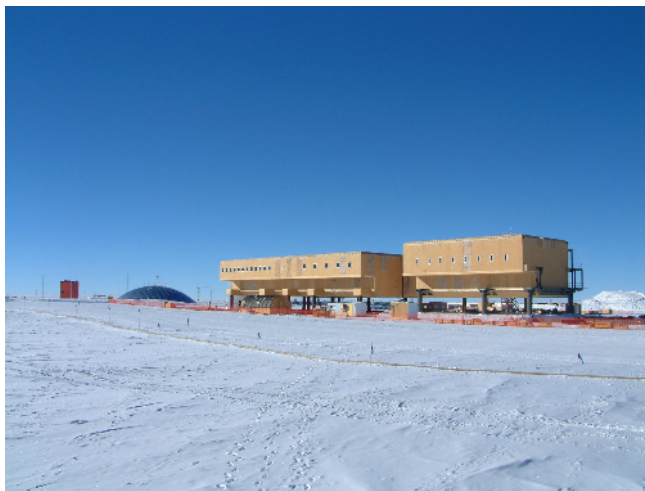
The isolated South Pole Station, currently under construction in Antarctica.
