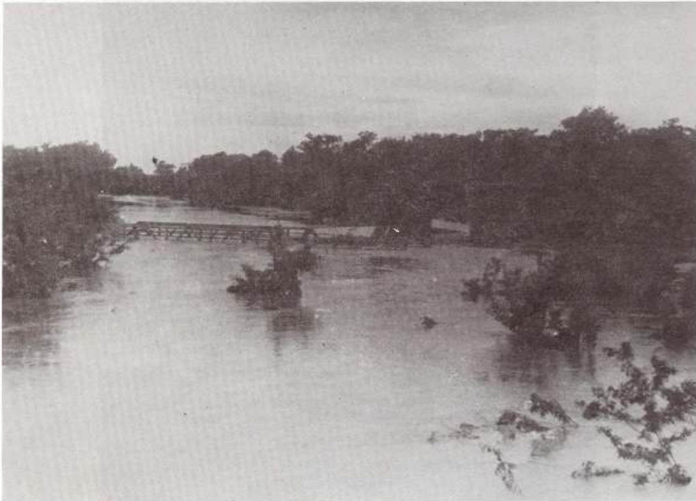
General Mouton Bridge (La. 729)
