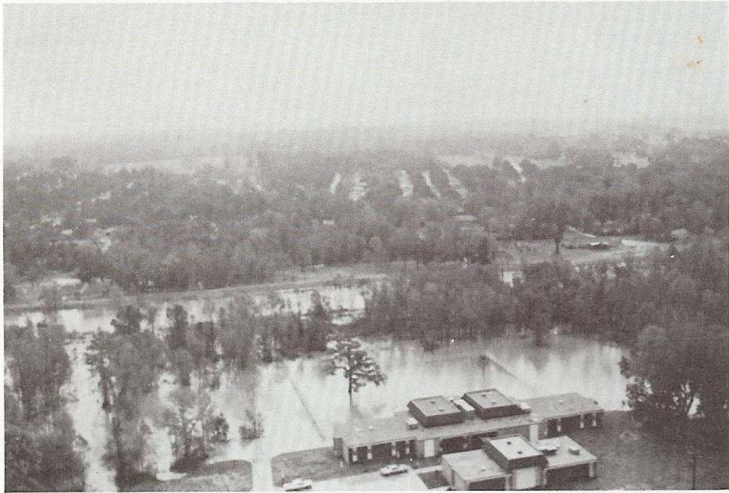
Detention home upstream of Surrey St. on the left descending bank.
