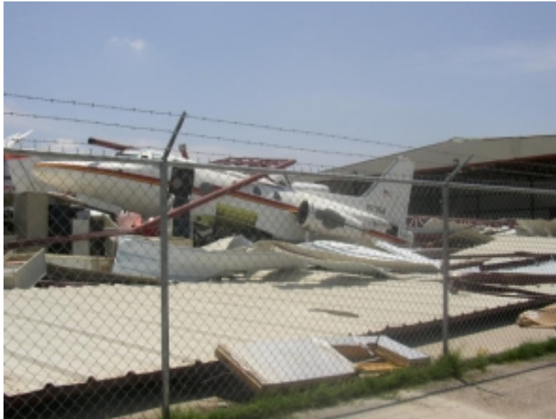
Four T-39 Saberliner Aircraft were destroyed inside hangar which failed under straight line winds. Picture was taken the next day at the Laredo International Airport.
