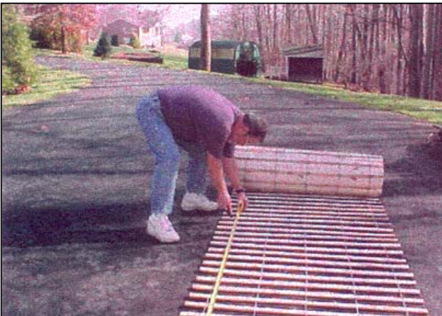
Picture 1: Snow fencing rolled out for measuring and cutting to length.
