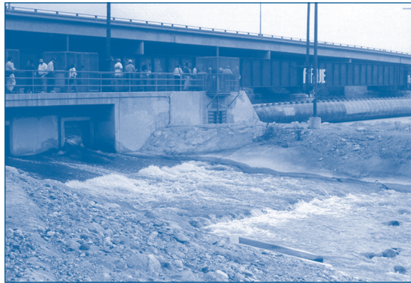
Field trip participants observe a release channel in the Santa Fe Spreading Grounds from a diversion headworks structure on the San Gabriel River. Photo courtesy Robert Dick, Natural Resources and Mining, Queensland Government, Australia.
