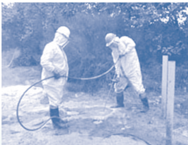
High-pressure remediation injection lance system for metals stabilization treatment.
