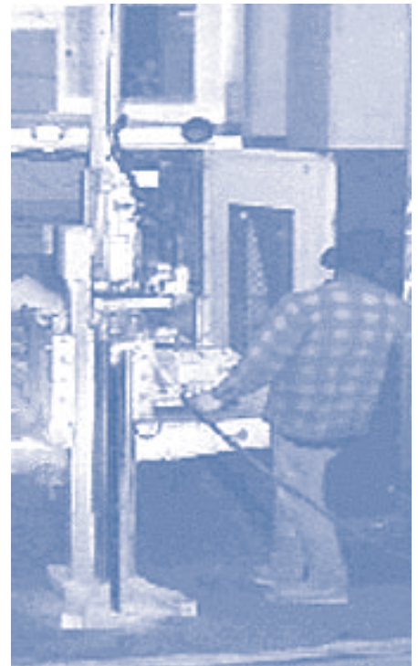
Installation of treatments liquids using the high-pressure Remediation Injection Process (RIP®)
