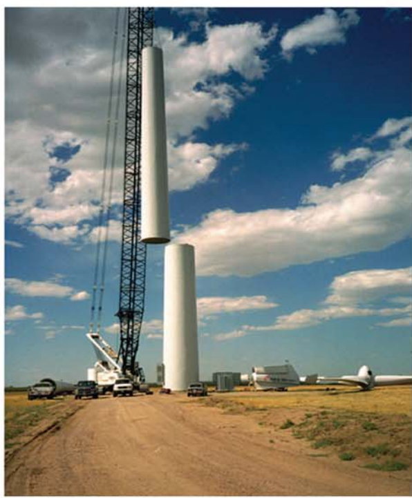
Turbine Tower Erection
