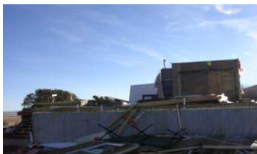
Ruby Valley , NV Wind damage Nov 2006
