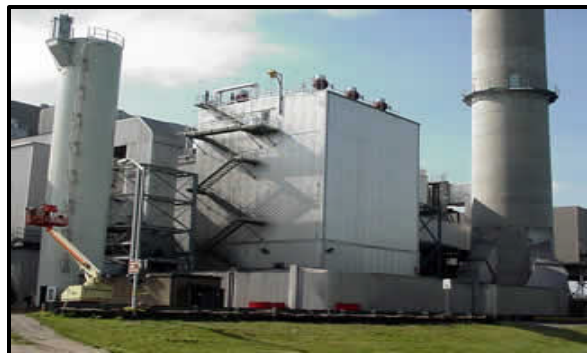
Figure 6-3. A fabric filter retrofit at a coal-fired power plant
