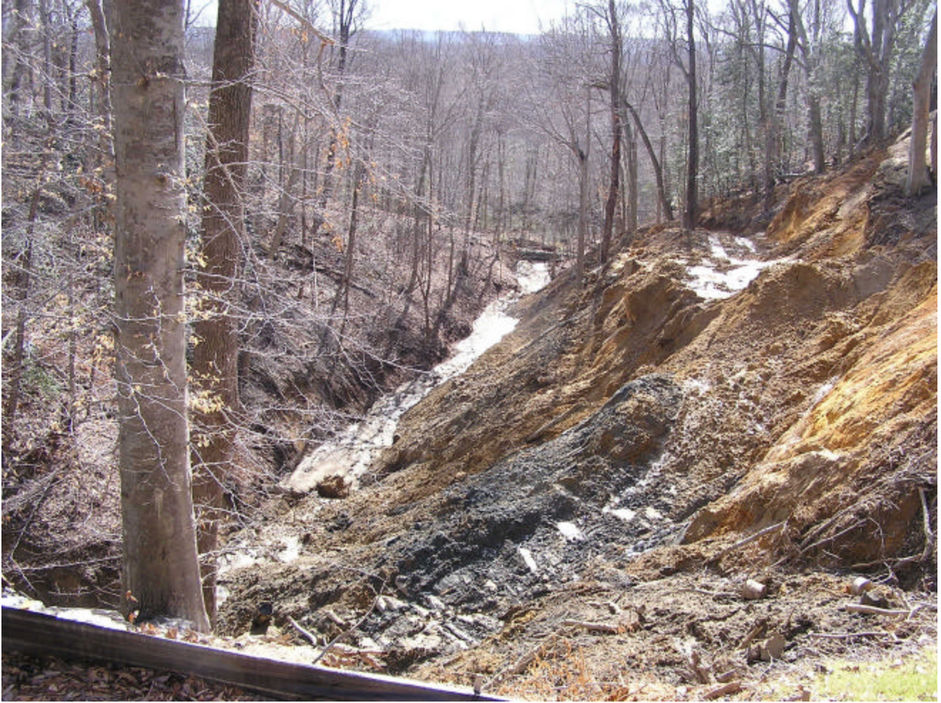
Lee Farm, after Tire Removal: Stabilization Still Needed
