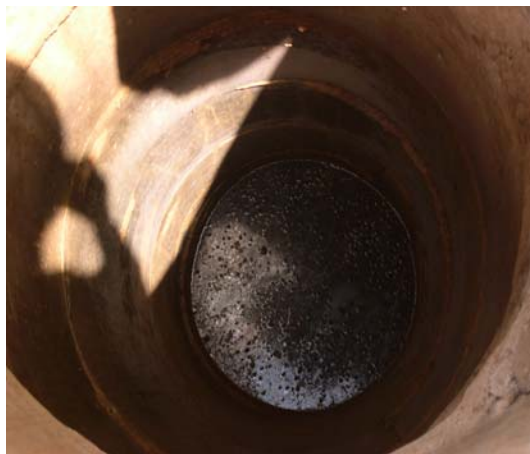
Resident's backyard well July 2005; water surface has oily sheen (EPA OIG photo)
